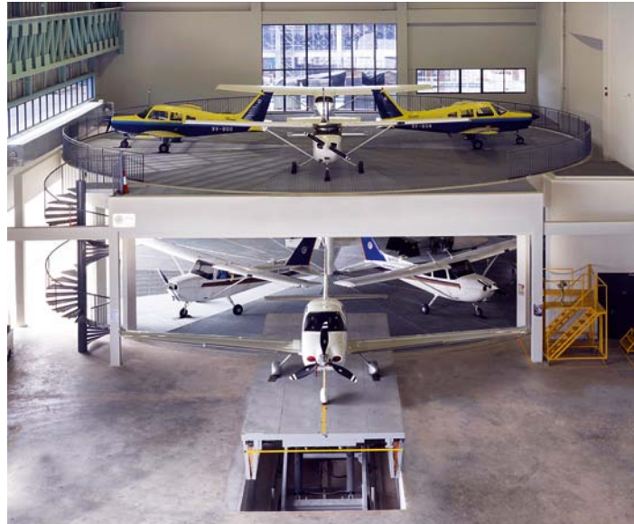
The latest award winning hangar design from Schaez Design and Construction is this multi level carousel system built in Singapore. Carousel hangars (multi or single level) save space, time, money and reduce hangar damage to aircraft.
