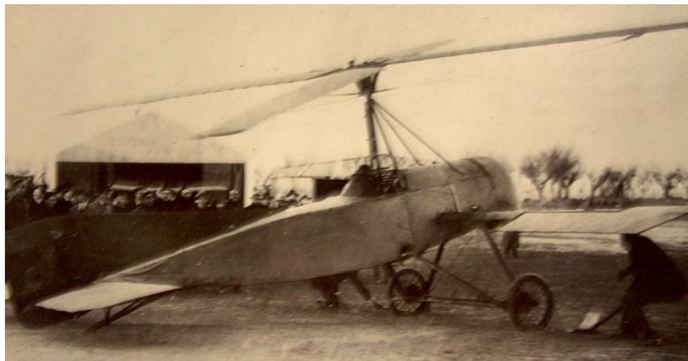
The Cierva C.4 was the first rotorcraft to make a controlled flight. Picture courtesy Dr. Bruce Charnov.
