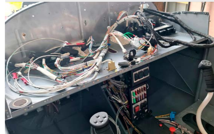
Wiring looms being prepared for the instrument panel.
