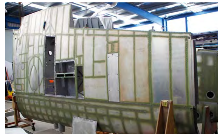
One of the wings well under way, the uncovered sections are for armaments.
