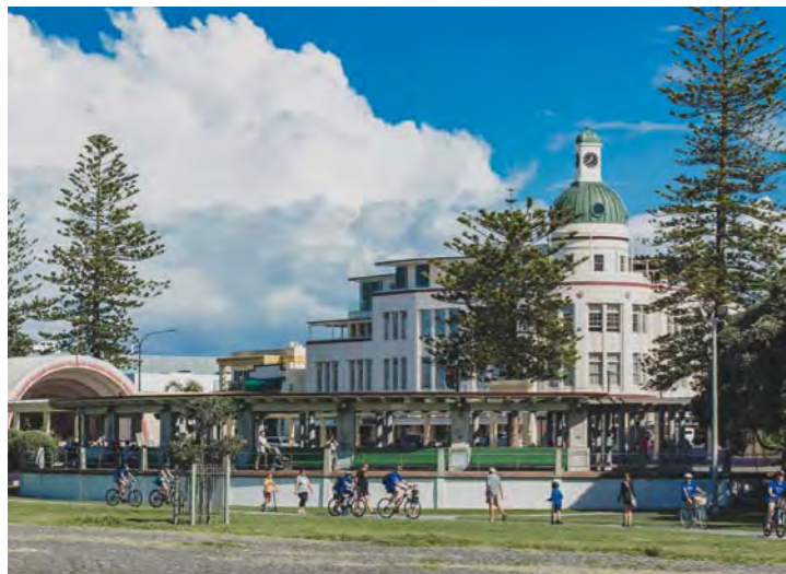
Napier's Sound Shell with the Temperance and General Building (1936) behind
